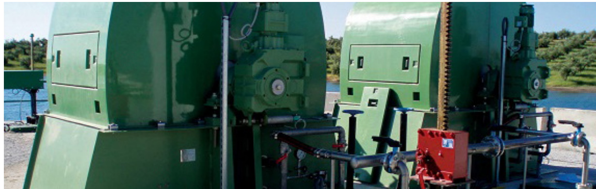
Geiger® Dual-Flow (Out-to-In-Flow) Travelling Band Screens
