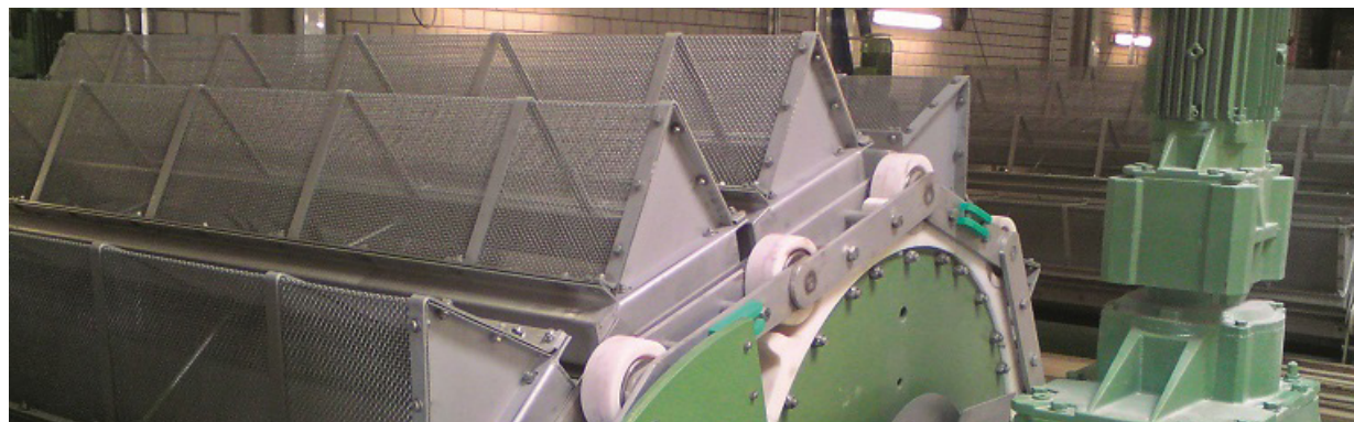
Geiger® Centre-Flow Travelling Band Screens
